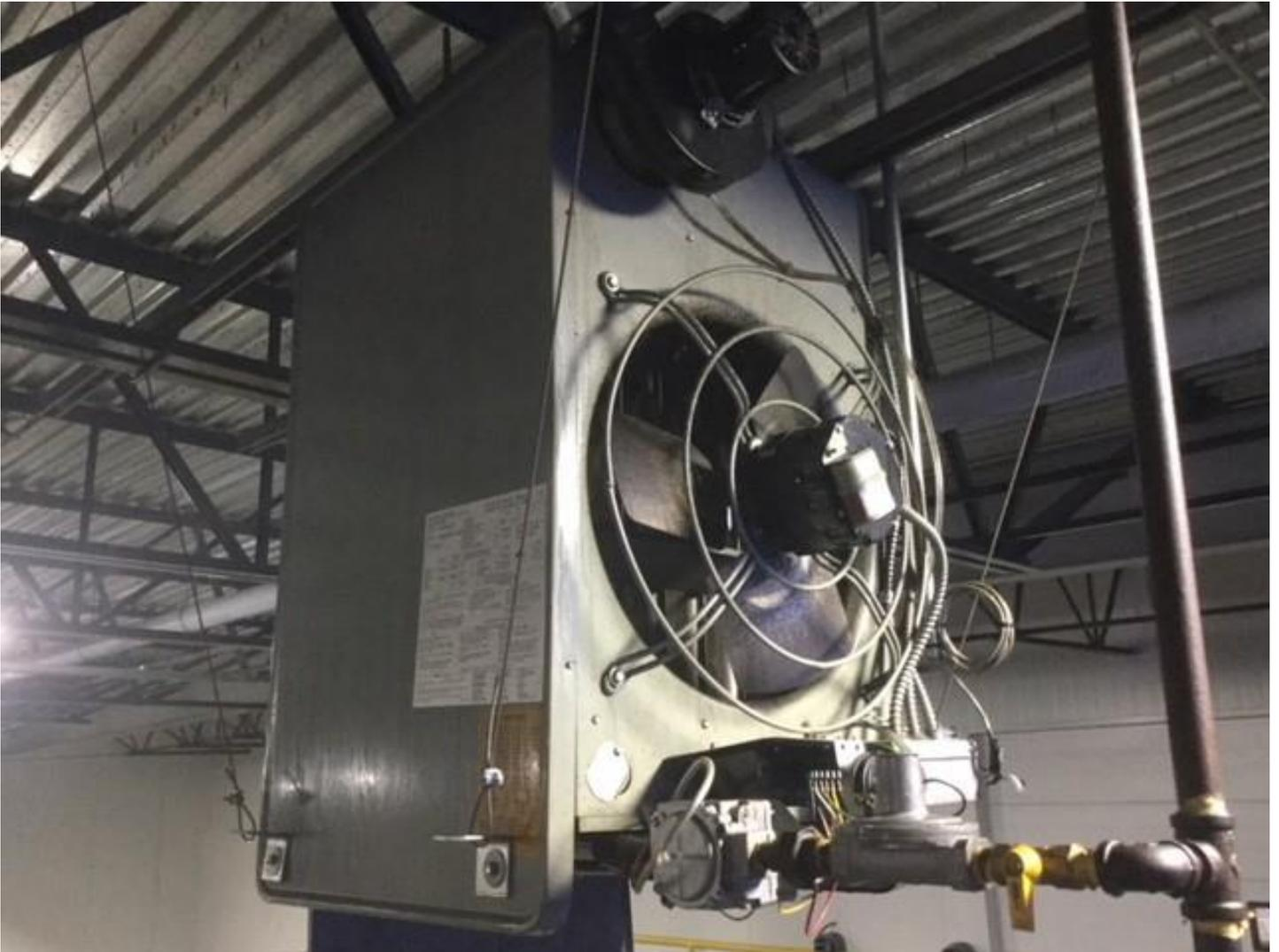
Pictured above is a typical warehouse heater (Unit heater) in normal working condition.
