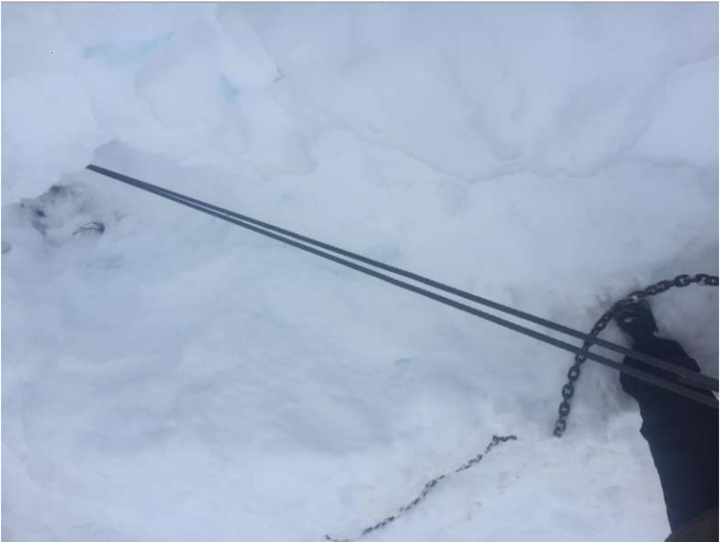
Tension Cable submerging into snow/earth connecting to buried anchor.
