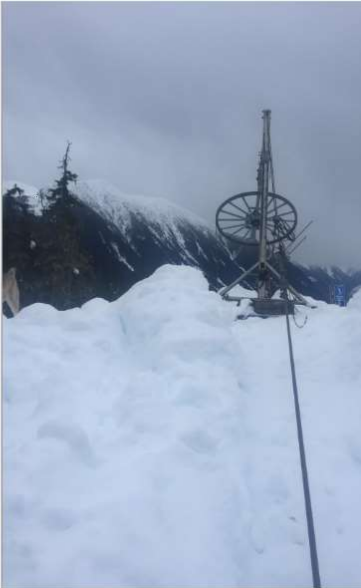
Station tilted forward due to anchor failure
