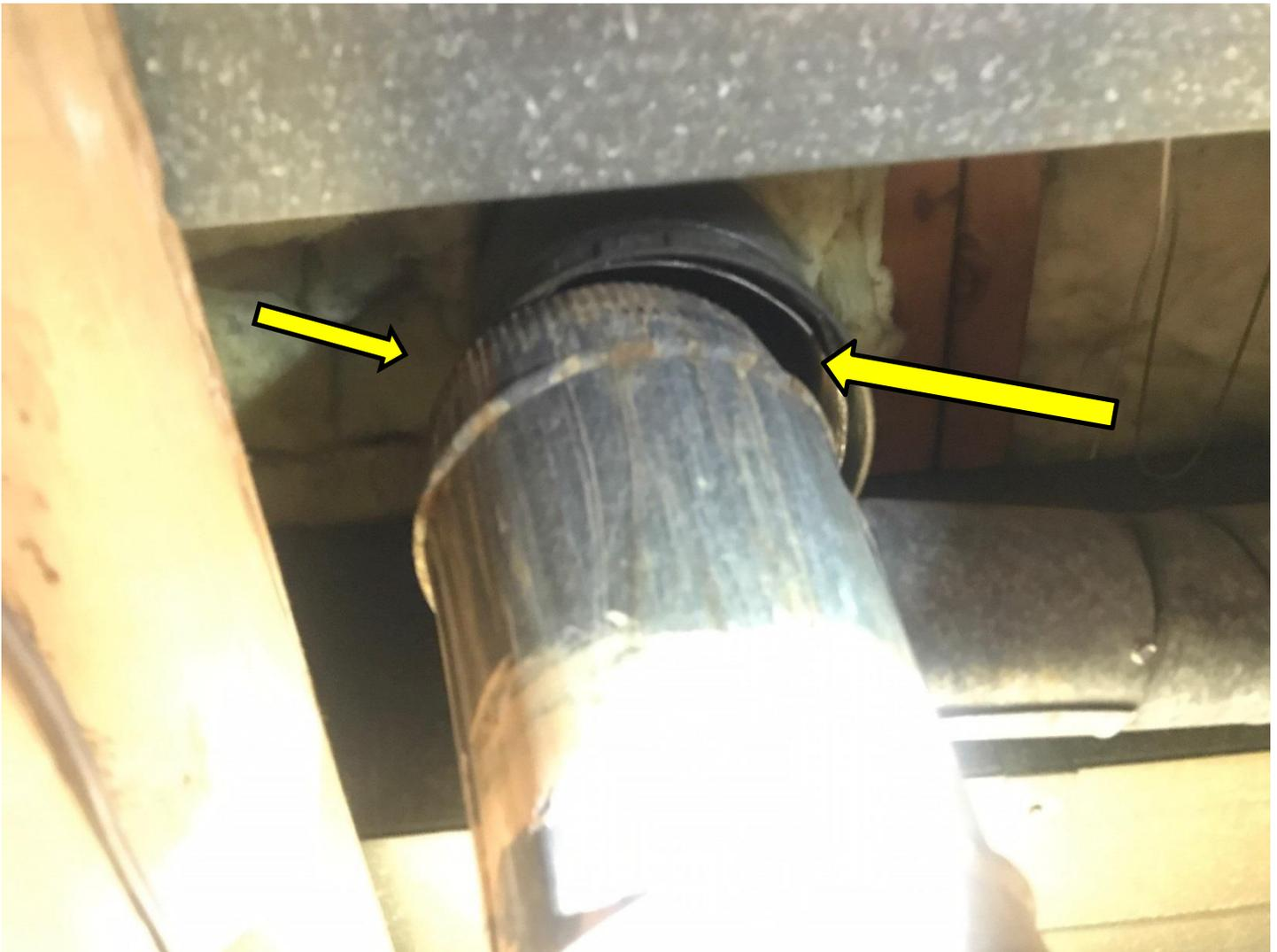
**Picture 1-** Yellow arrows point to where flue gasses were spilling from dislodged vent. Horizontal section of vent is where water heater is connected into furnace vent.
