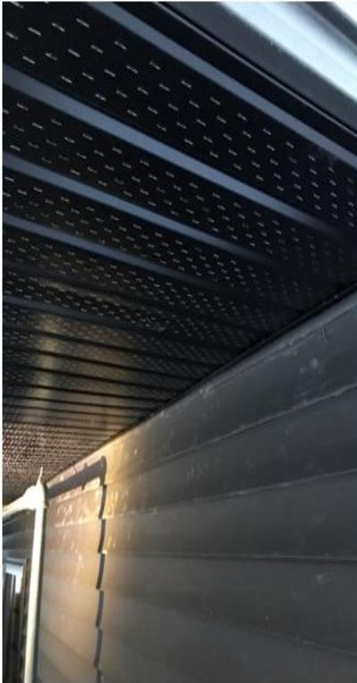
**Hole cut in soffit shows building air intake.**
